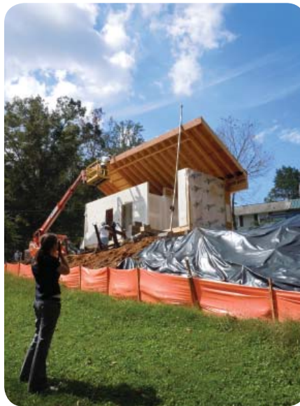
Incomplete modular units are delivered to site for custom interior and exterior finishes. (left) View of finished interior of the home. The marriage wall acts as the primary organizer of spatial functions. (right)
