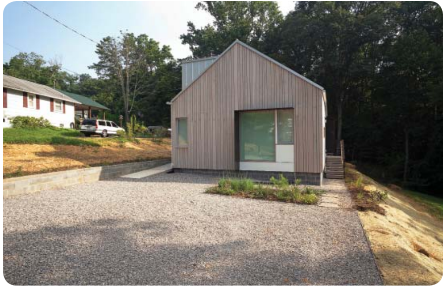
View of parking court and south facade of home. (above)
