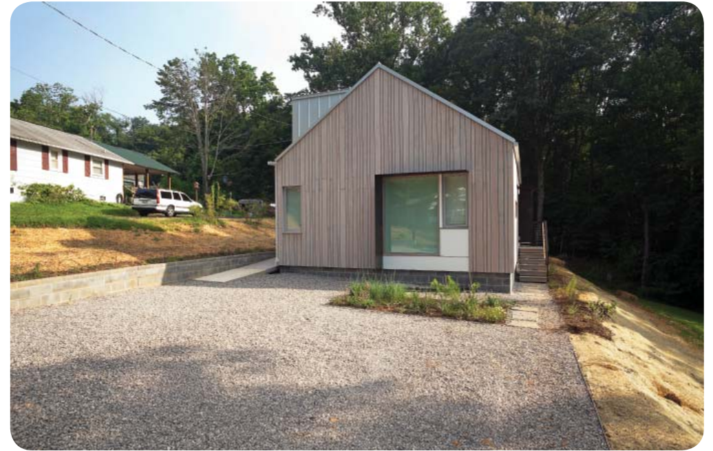
View of the parking court and home from the street. The home is clad in Atlantic White Cedar, a regional material chosen for its natural resistance to moisture damage and weathered grey appearance. The steel canopy provides functional shading to southern glazing, but also acts as a formal element in the composition of the façade. (above)
