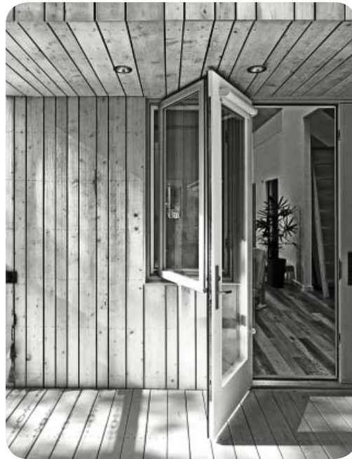
French doors in the rear of the home extend the living space into the landscape. I was responsible for the design and detailing of the soffit, which is clad in Atlantic White Cedar and creates a sense of continuity between the two planes. (above)
