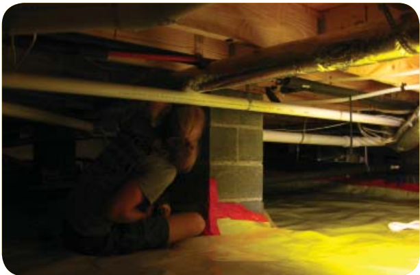
Foundation detail showing radon resistant construction techniques. The crawlspace has been covered with 12-mil polyethylene sheeting (exceeding the minimum 6-mil set forth by the EPA). (above)
