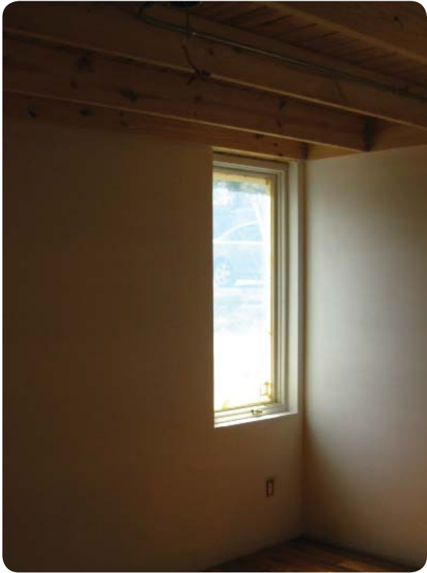
Modular units are set on-site 24" O.C. roof joist spacing (top-left)
