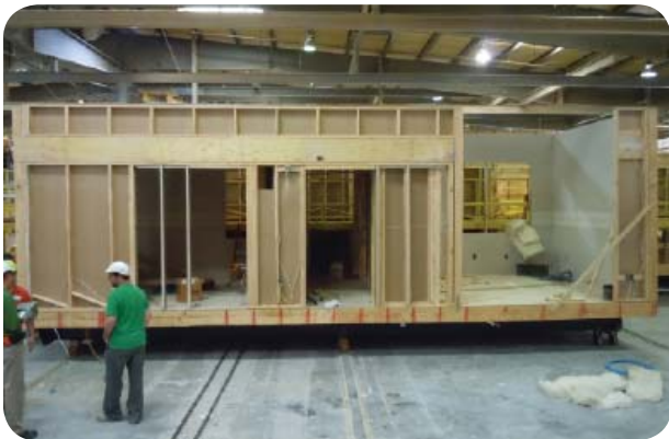
“Interior Board” is applied to marriage wall in Bean Station facility. (above-left)
