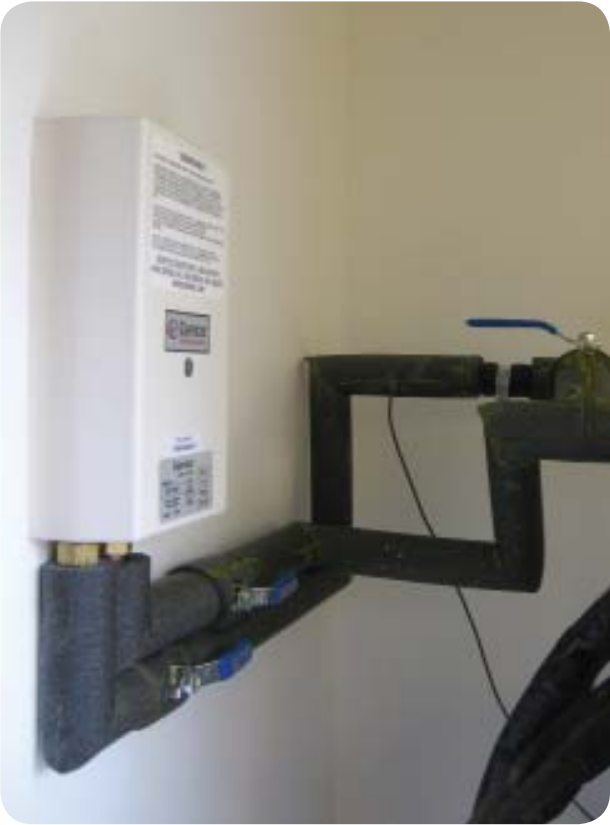
All hot and cold water lines were pre-insulated at Clayton Homes manufacturing facility (left)
