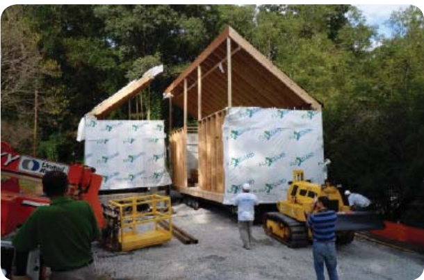
Interior walls are installed in modular unit. Rough electrical and plumbing work has already been stubbed out of the floor. Exterior walls are applied next. (top-left)
