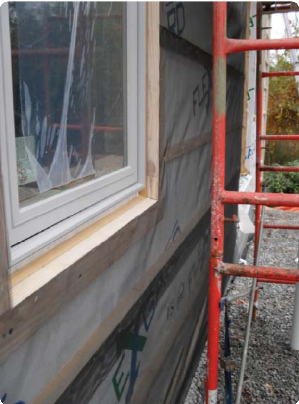
A typical operable window condition with all external cracks and joints adequately sealed (top-left)
